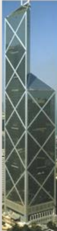
Similar cross bracing seen on the Bank of China
